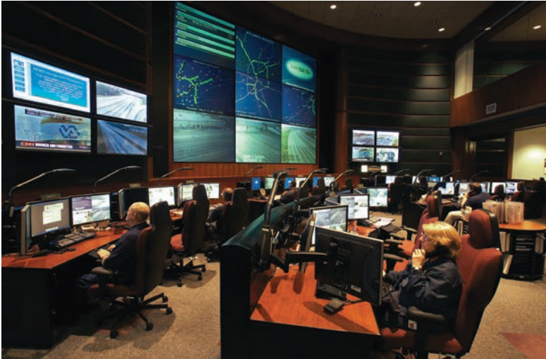
At the Georgia Department of Transportation, single-tier Profile consoles were configured in a 15° concave fashion providing clean sight lines to wall-mounted plasma monitors and a central video wall.
