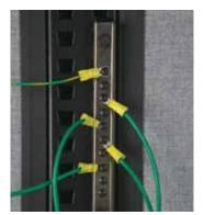
**ESD Controls**Common point ground bar.
