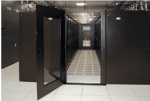
Cold-aisle containment
